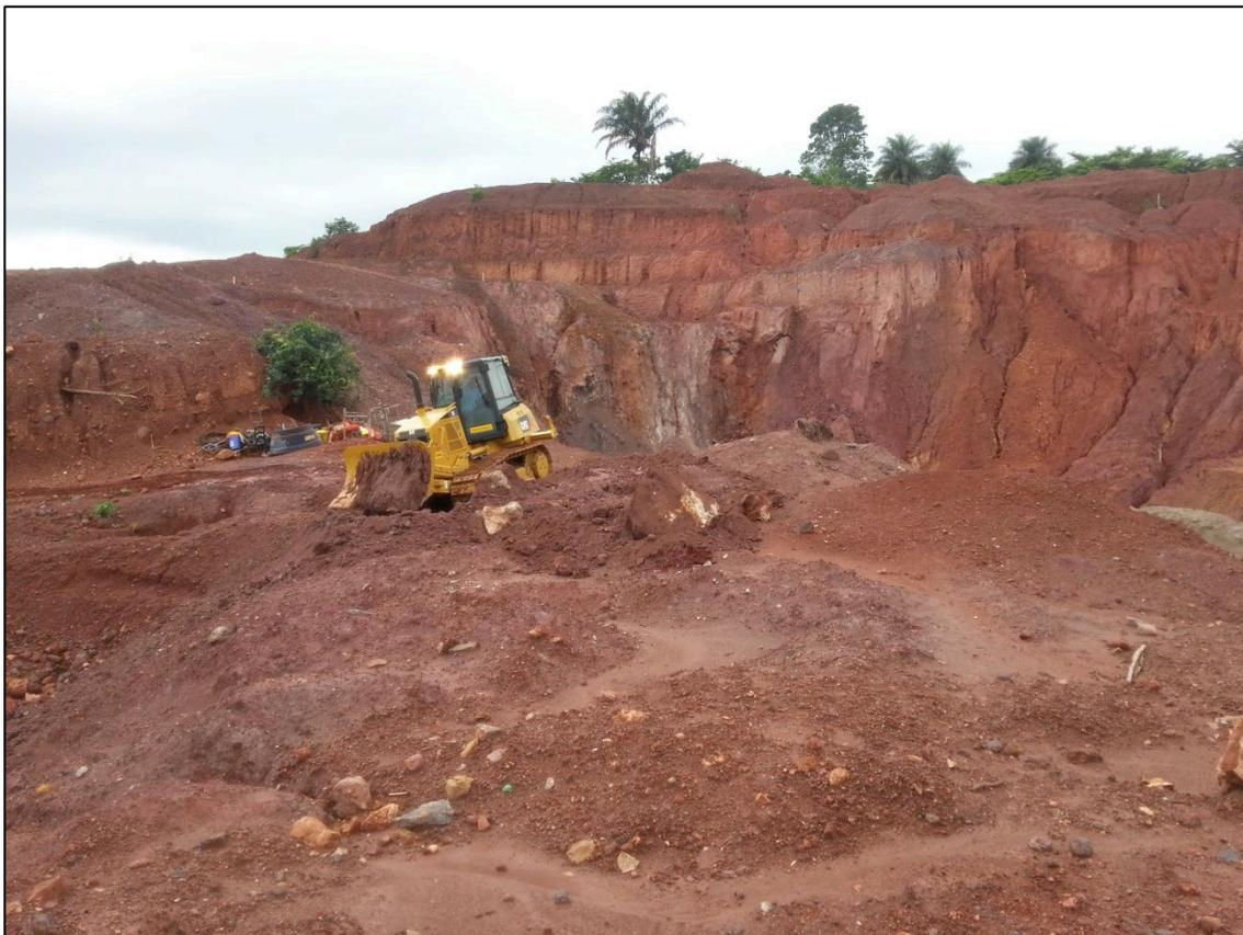
Photo 6 - Bulldozer preparing a drill site at the Osmar Target.
